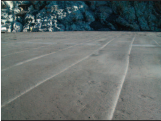
Typical aspect of the surface of a compacted "RCC-friendly" mix, referred to by Ibáñez de Aldecoa.
