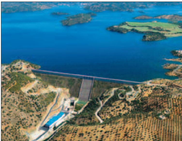
View of La Breña II RCC dam (119 m high, with an RCC volume of 1.44 \times 10^6 \text{ m}^3 ) completed in 2008 in Spain. It is the largest RCC dam in Europe.
