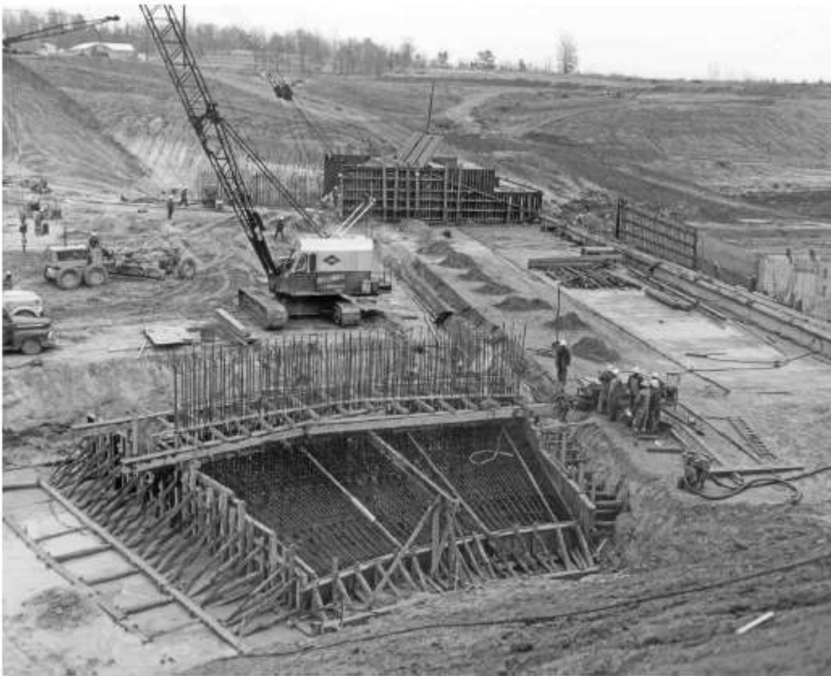
Figure C.6 – Photo looking east at construction of uncontrolled spillway.
