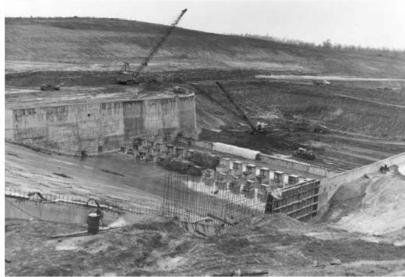
Figure C.4 Photo looking east-southeast at partially completed spillway stilling basin.
