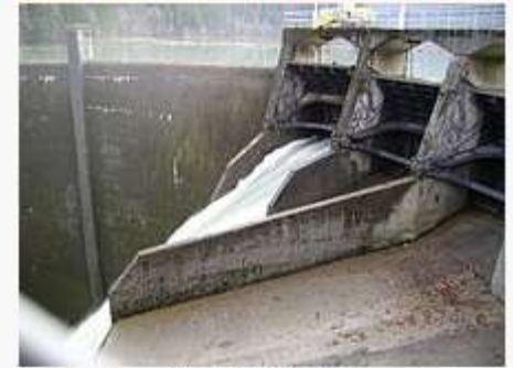
Glines Canyon Dam
